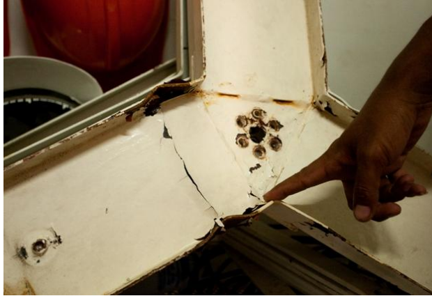
Fig. 2 Photograph of a damaged turbine blade bracket caused by large flapwise bending moment during a horizontal gust (taken at the wind farm on Koh Larn, Chonburi in June 2009)
